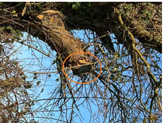
T11 – Flush-cut with no visible cavities
