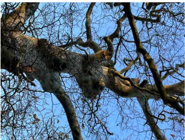
T29 – Knotholes throughout, some extending
