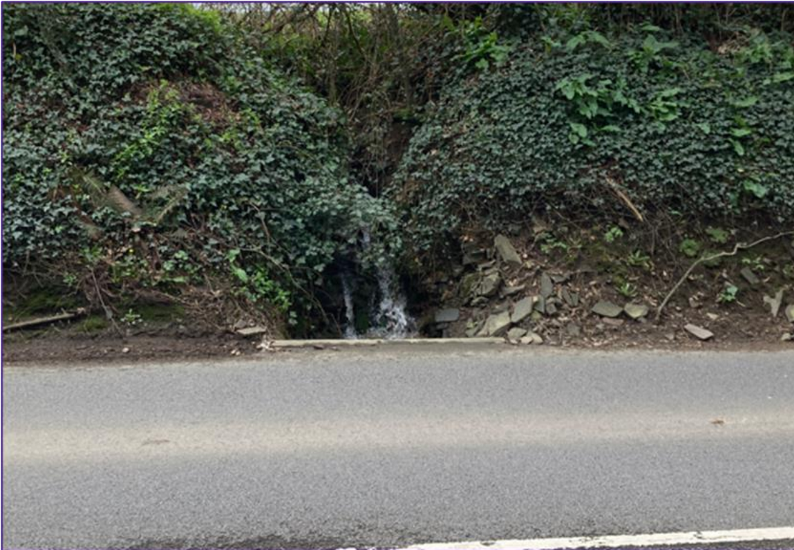
Plate 1.6: Culvert which runs under the A386
