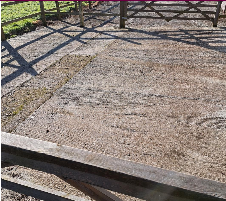
Plate 25: Area 3 – Hardstanding Around Farm Structure (SE)
