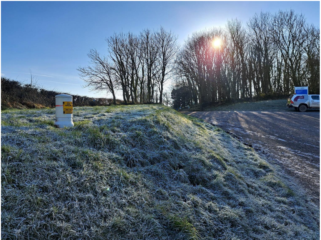
Plate 18: Western Road, Site Access Gas Pipeline Marker (SE)
