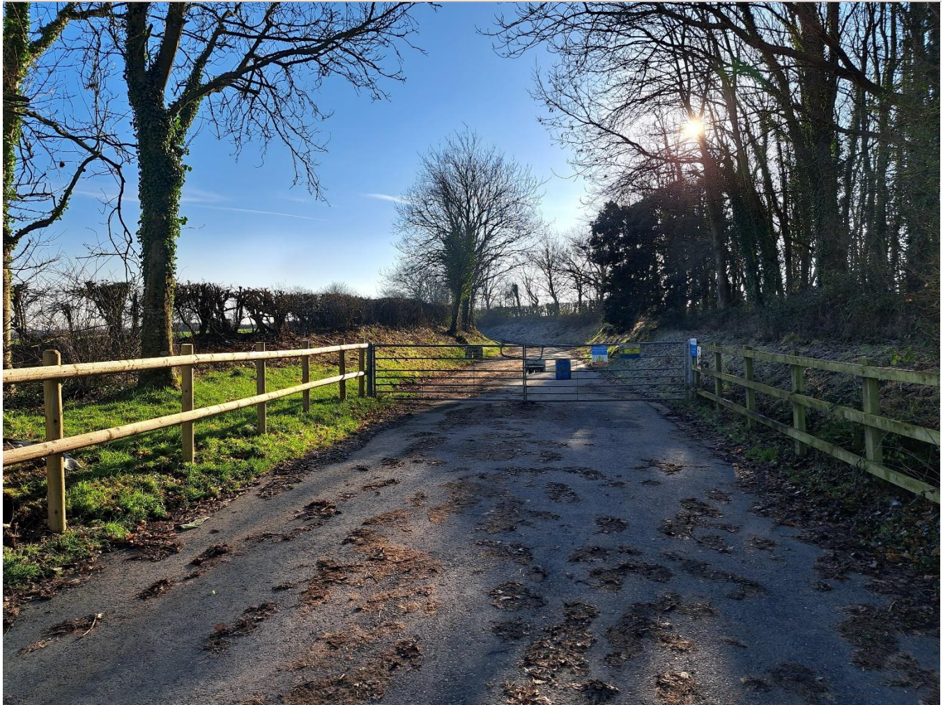
Plate 1: Entrance Road to Alverdiscott Substation (E)
