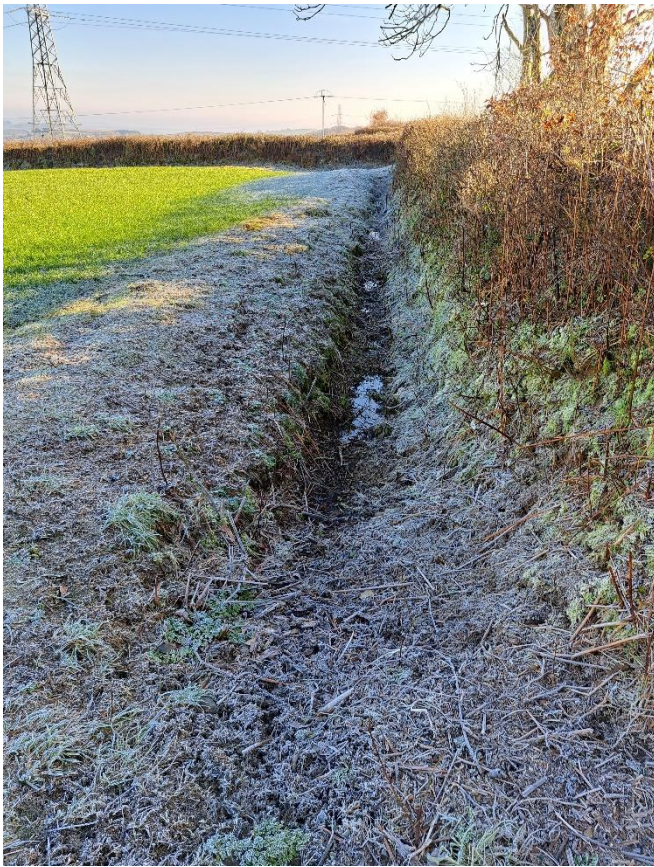
Plate 14: Area 1 – South Boundary Ditch (E)
